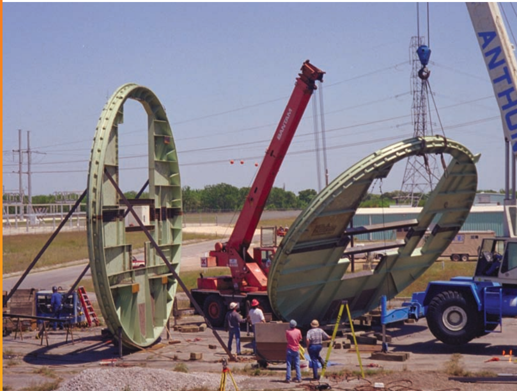
Assembly of rotary dumper.
