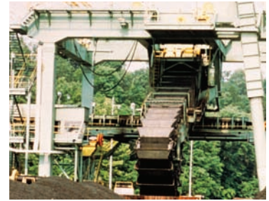
Mechanical and Electrical Upgrades
