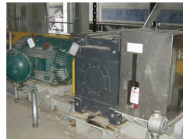
Drive With Disc Brake Option
