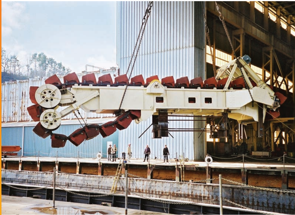
Barge Unloader Boom Replacement
